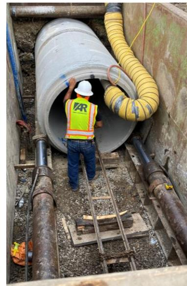
for the bell end of the pipe. Approximately 1,200 cubic feet of soil were excavated to create the 223' double barrel pipeline that runs approximately 16 feet below top of grade. All the excavation of soil for this project was removed by hand. The pipe diameter, length of run, ground conditions and other factors were carefully considered when determining how much thrust should be used to jack a pipe through the soil.
