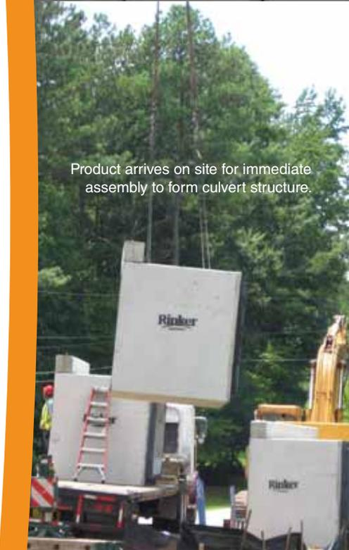
Product arrives on site for immediate assembly to form culvert structure.
