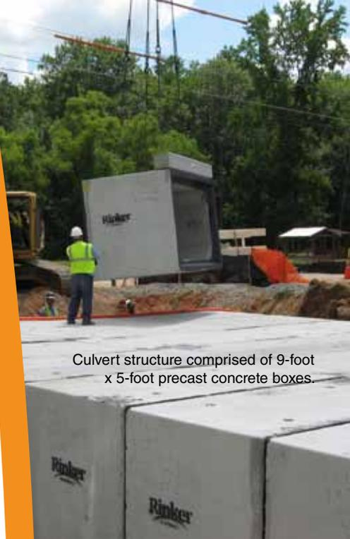
Culvert structure comprised of 9-foot x 5-foot precast concrete boxes.
