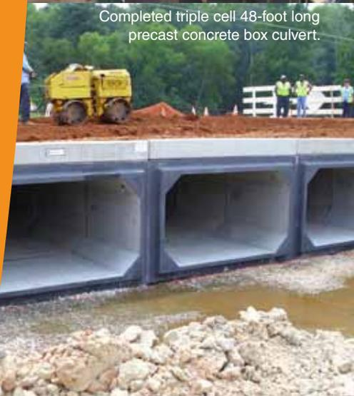
Completed triple cell 48-foot long precast concrete box culvert.
