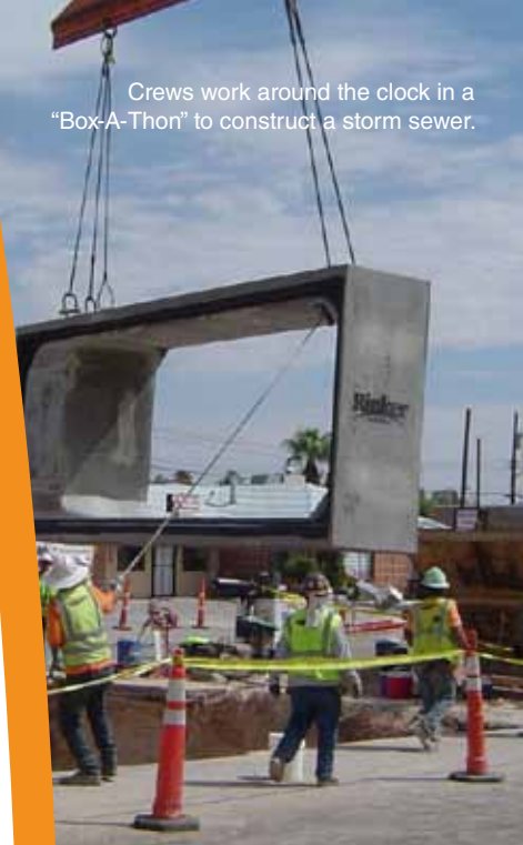
23-foot x 8-foot boxes were the largest ever produced using a drycast method.
