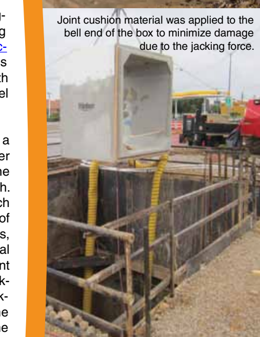
Jacking against a reaction block in the launch pit.
