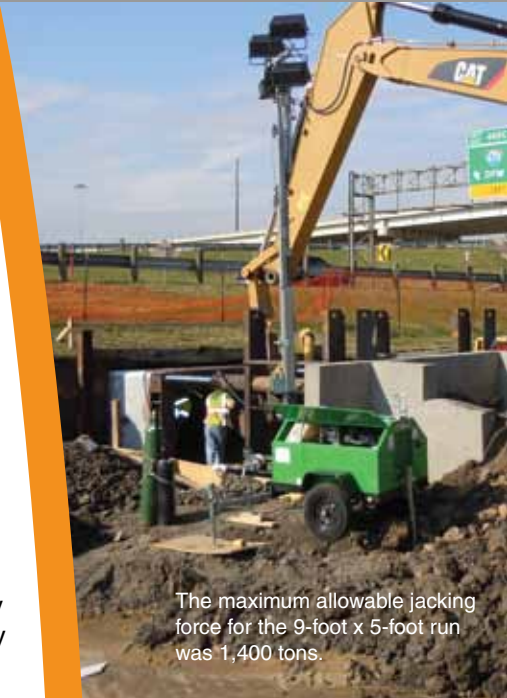
Joint cushion material was applied to the bell end of the box to minimize damage due to the jacking force.
