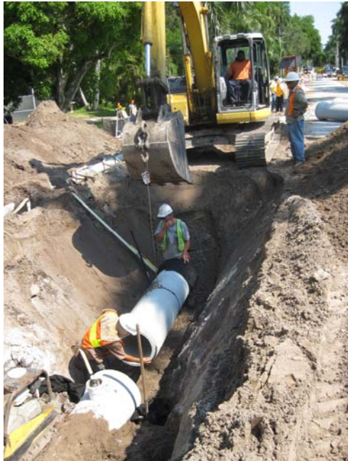
Figure 3. RCP joints were efficiently installed and tightly homed.
